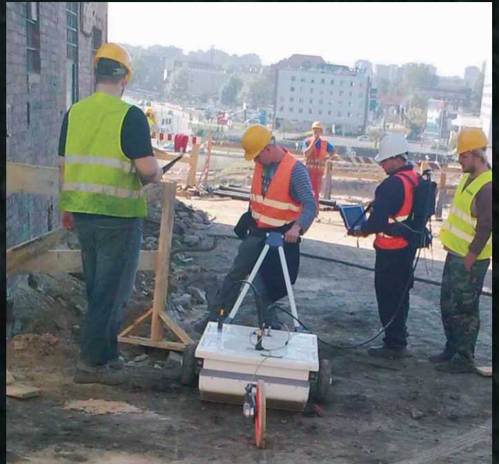
Georadar acquisition to identify the structure of the soil, geotechnical borders and cracks in the rock during construction.
