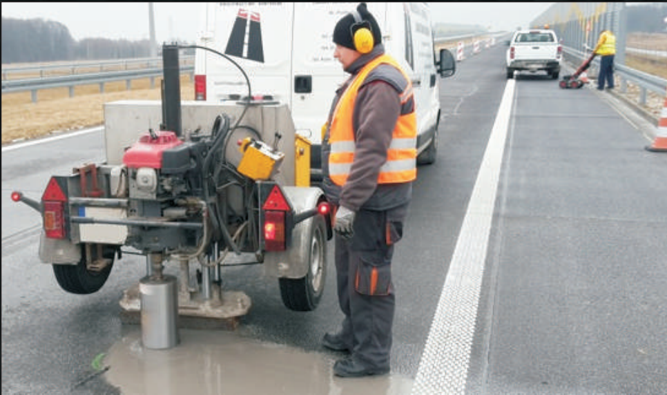
Mechanical drilling in concrete layers on highway, located in place of observed and marked cracks on surface (top) and a core of two outer layers of concrete separated by a geotextile, with a visible long vertical crack in top layer (right).
